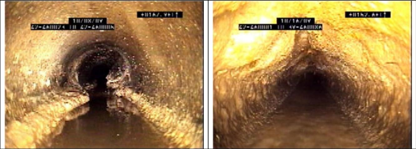
Grease buildup is the most common cause of gravity system sewer lateral and main line backups. A gravity system operator communicates basic guidelines to help slow the
